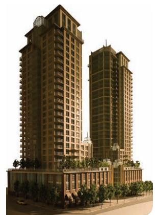
Construction starts this fall on Vita, the first tower of Symphony Place, at Richards and Smithe.
